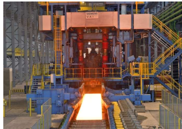
Roughing Mill with Edger
