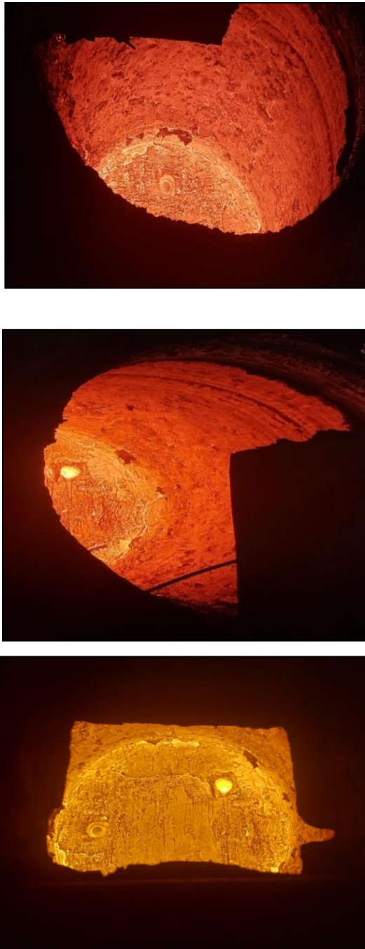
Figure 13: Ladle Lining Conditions after 148 th Heat
