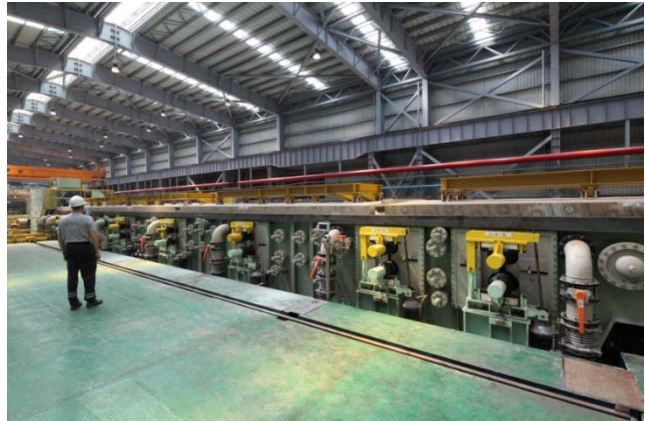
Fig 7 High-tech continuous Turboflow® Pickling Section
