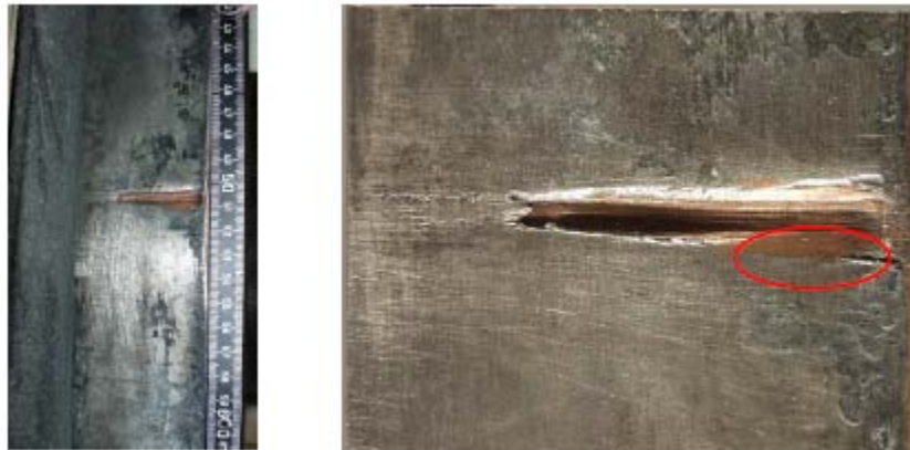
Fig 8 Narrow face plate with damaged edge at the corner by hard particle 7
