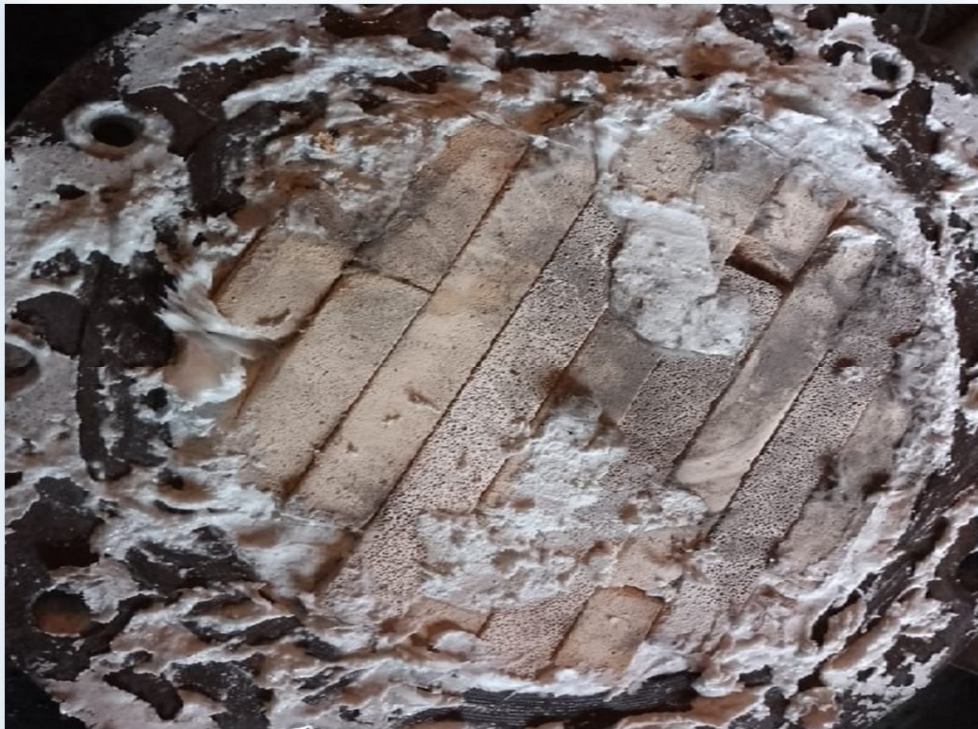
Surface of the brick structure
