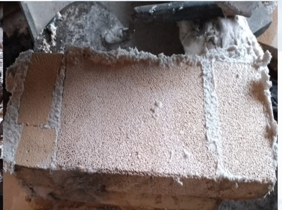
Inside the brick structure
