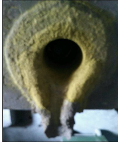
Induction Slag Furnace (top view) after lining
