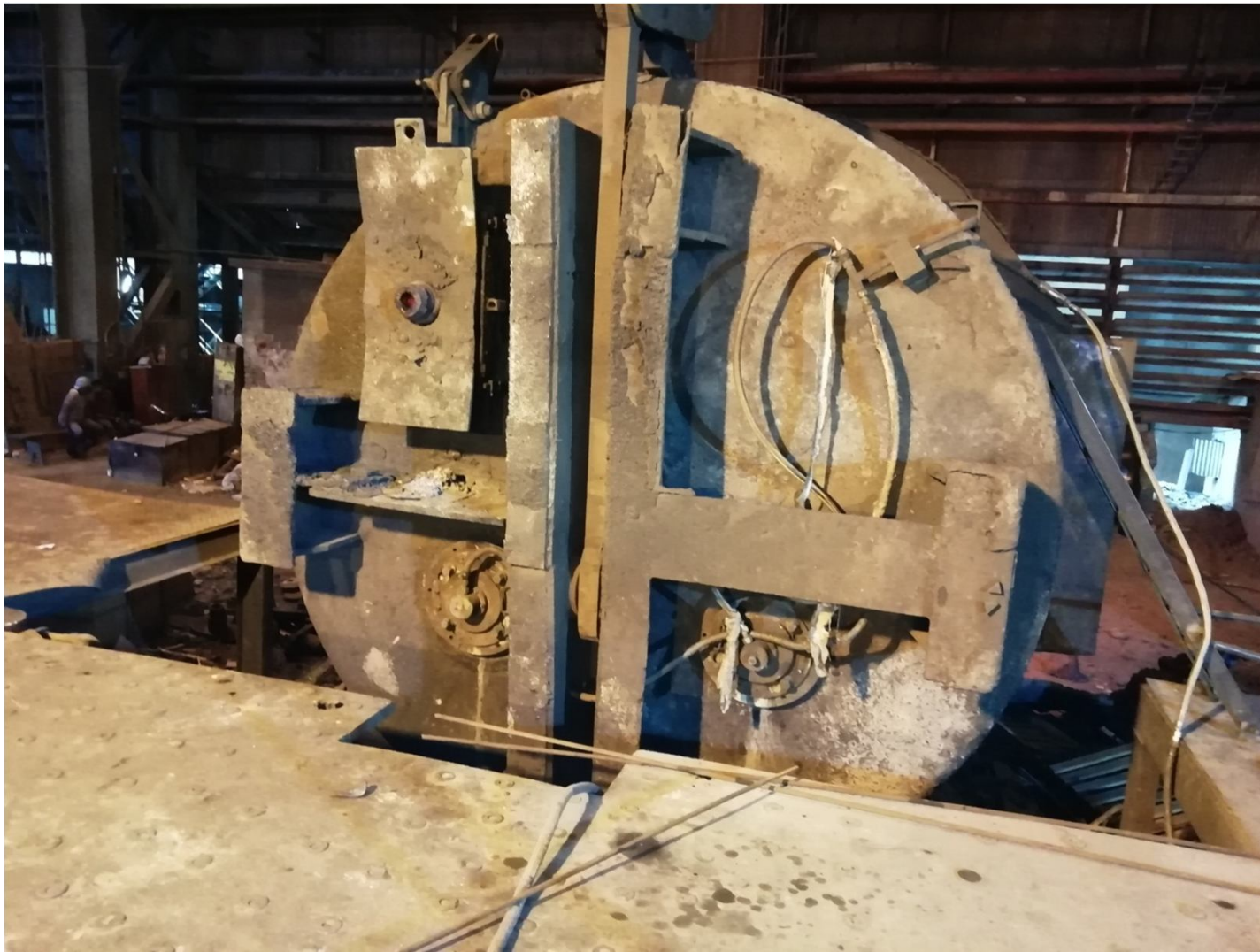
Modified Steel Ladle with both Porous Plugs at Durgapur Steel Plant
