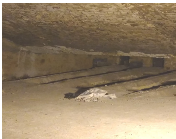
Figure – 1: Final condition of preheating zone hearth after refractory lining
