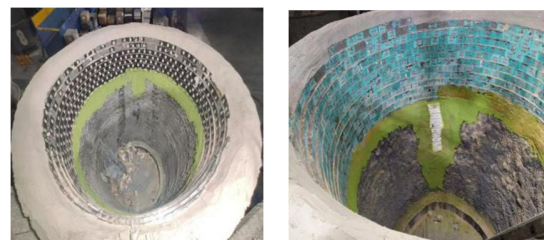
Fig 5: Ladle during repairs
