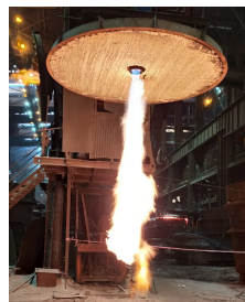
Figure-2: Flame of newly designed burner
