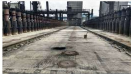
Oven Top Maintenance
