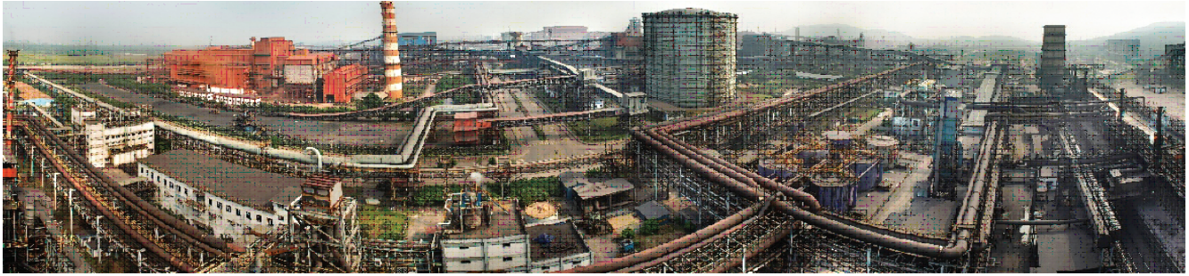
Tata Steel Kalinganagar plant, Odisha
