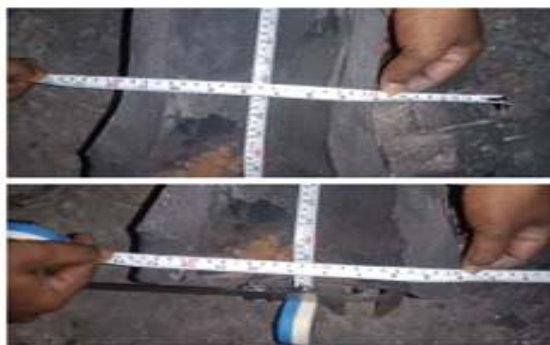
No Air ingression , internal erosion , liner intact
