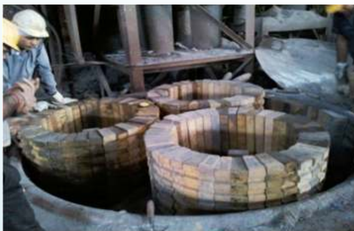
Figure – 1: Refractory lining of EAF roof is in progress
