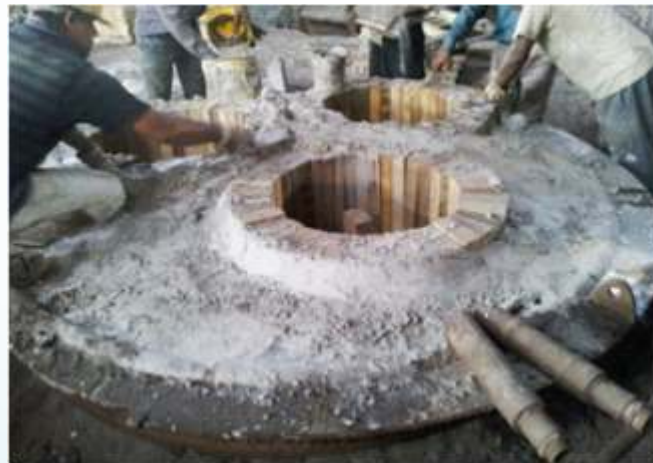
Figure – 2: Final stage of EAF roof refractory lining
