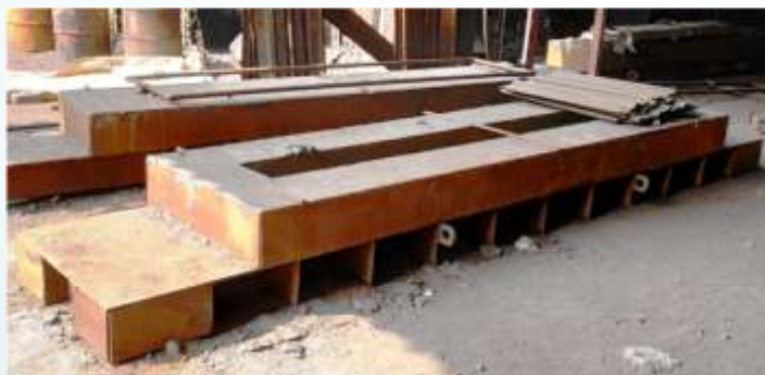
Figure 8 : Precast prefabricated new refractory beams for burner
